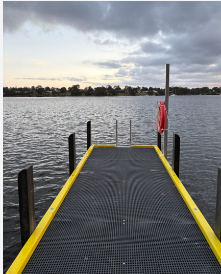
Full FRP Jetty Rebuild – Sunset Cove, Paynesville
